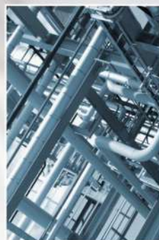
Heating equipment inspection
