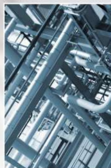
Heating equipment inspection
