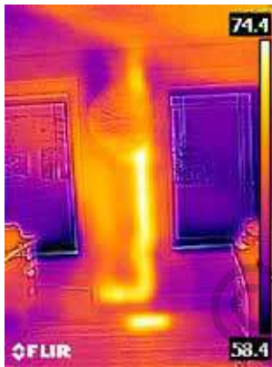
Warm drain pipe in wall
