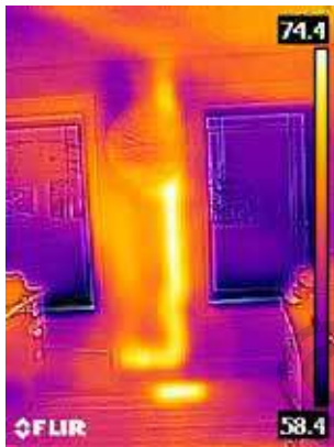
Warm drain pipe in wall
